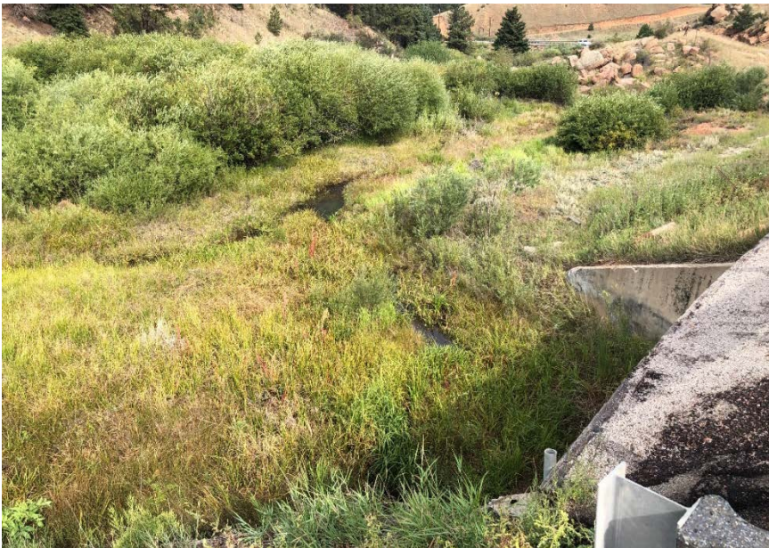
Photo 4. Avoidance Area 4 consists of the wetlands, tributary to Twin Creek, and main channel of Twin Creek located around Bridge I-15-AO, another bridge associated with the Region 2 Bridge Bundle project. The full wetland and OHWM delineation can be found in the I-15-AO Aquatic Resources Delineation Report.
