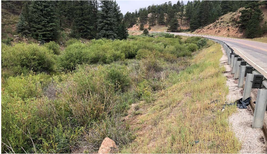
Photo 1. Avoidance Area 1 (AA1) consists of a stretch of the main channel of Twin Creek that is located within the PRA but outside of the PIA.
